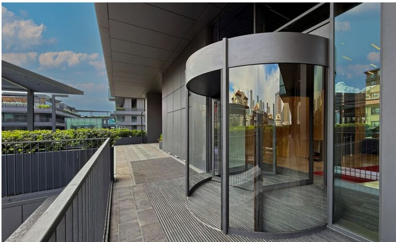
Manual revolving door system for three- or four-leaf doors
